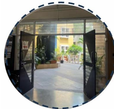
MAIN DOOR (INSIDE)
