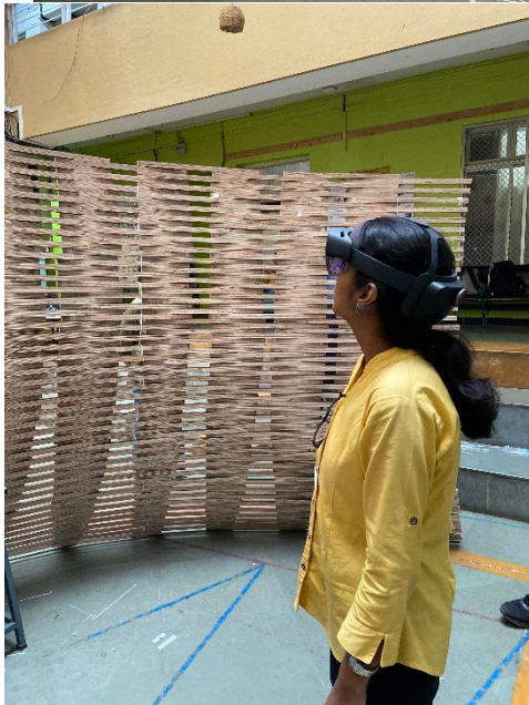
Students physically stacking the assembly with the help of Microsoft hololens
