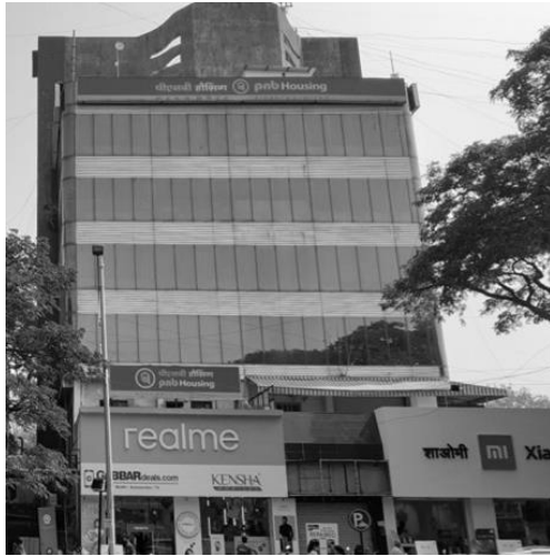
Fig.3. Glass facade building.
