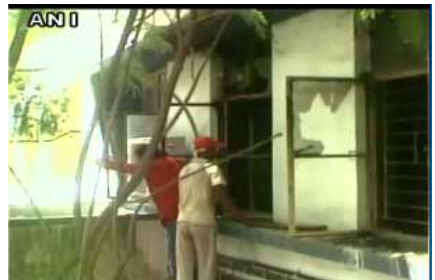
Fig. 4: Patients break windows to escape from Govt hospital in Murshidabad 6
