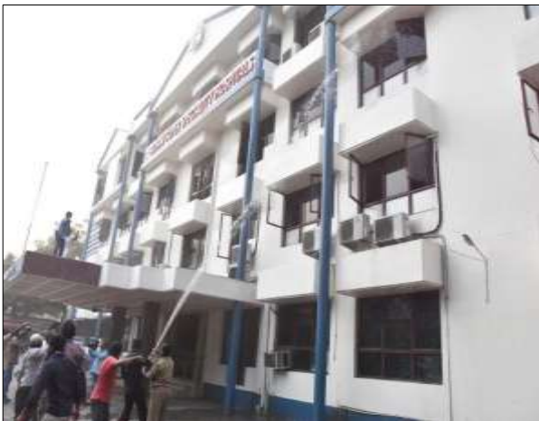
Fig. 3: Fire fighters dousing the fire during the rescue operations at Rohini hospital in Warangal 16 .
