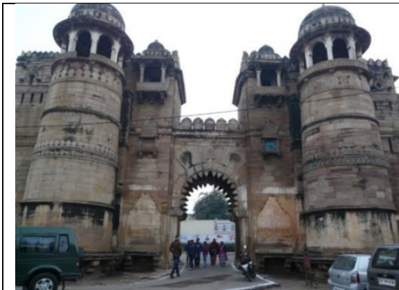
Figure 13: Entrance Gwalior fort
