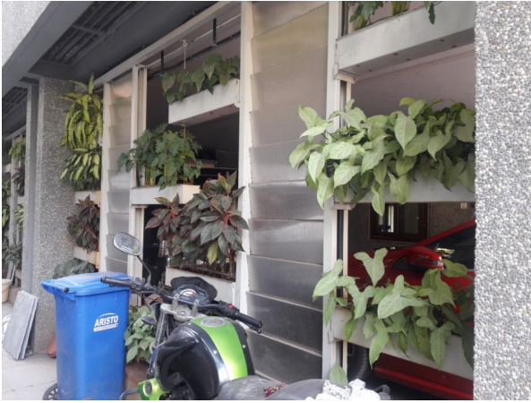
Figure 5. Intermittent panels of water systems along with vertical gardening cooling the internal rooms
