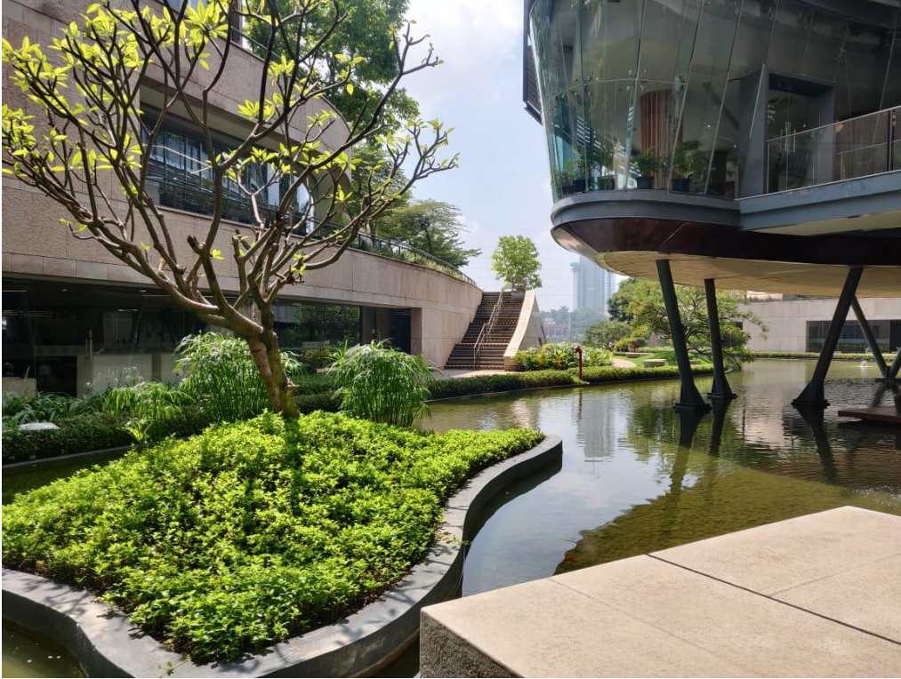
Titan Integrity Campus
