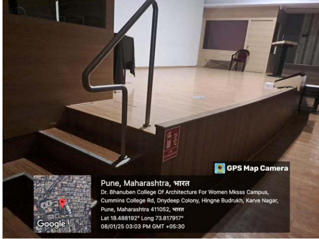
Railing at auditorium stage at BNCA
