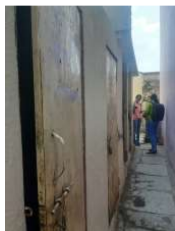
Fig 03 – Existing Boys Toilet
